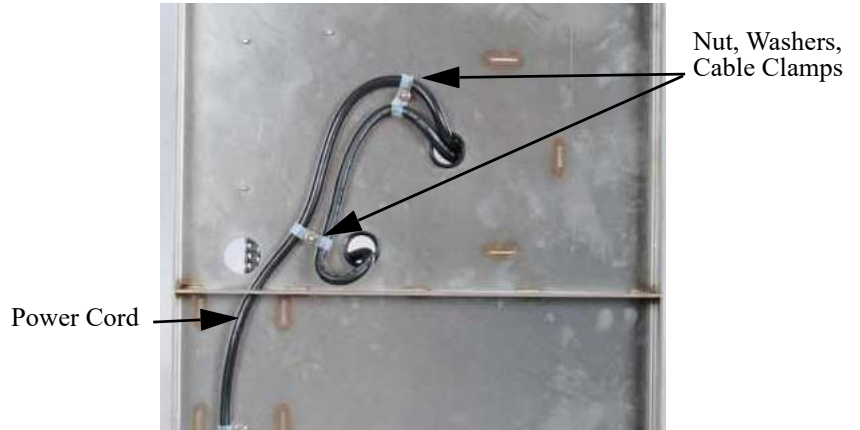
Underside Of Frame
