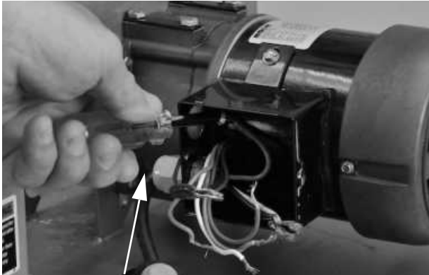
Motor Cord installed in the bottom hole of junction box
